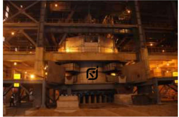
TATA STEEL LTD. GOPALPUR. - 2 Nos. 18 MVA
