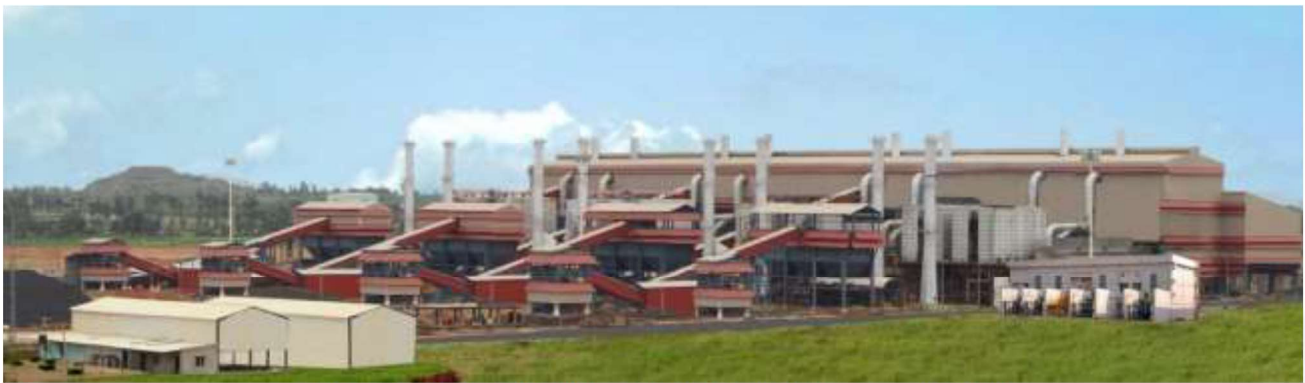
ABHIJEET FERRO TECH (P) LTD., VISAKHAPATNAM 8 Nos. 22.5 MVA
